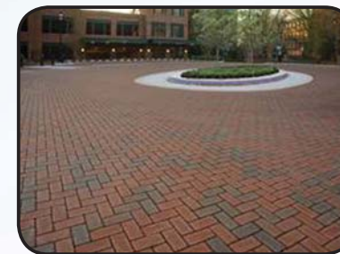
Permeable Pavement in Pedestrian Access Areas, Gott's Court, Annapolis, MD
