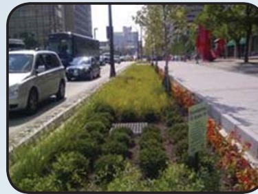
Micro-Bioretention, Baltimore Inner Harbor
