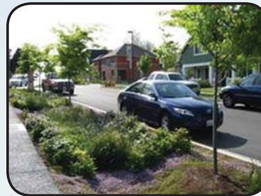
Bio-Swale, Seattle, WA
